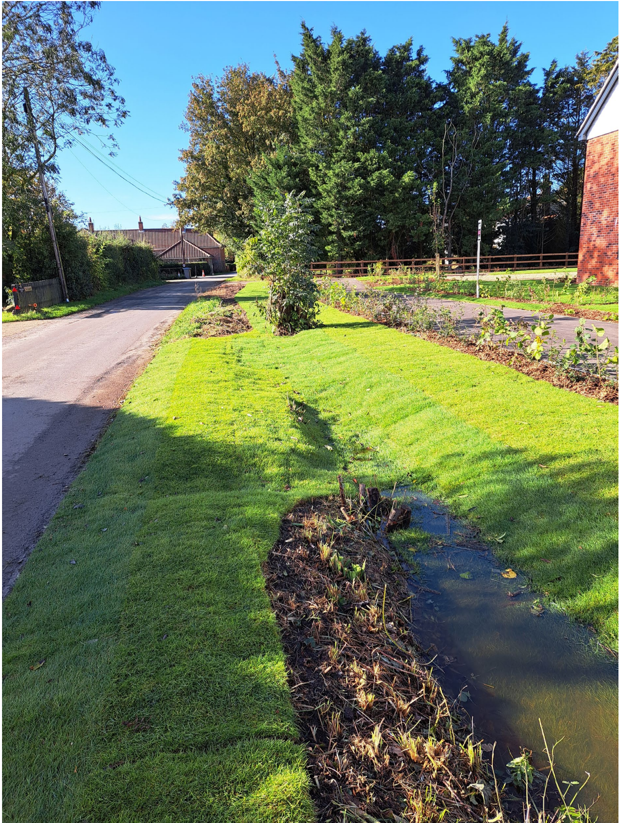
14 October 2023. End of remaining part of ditch and filled-in part of ditch.
