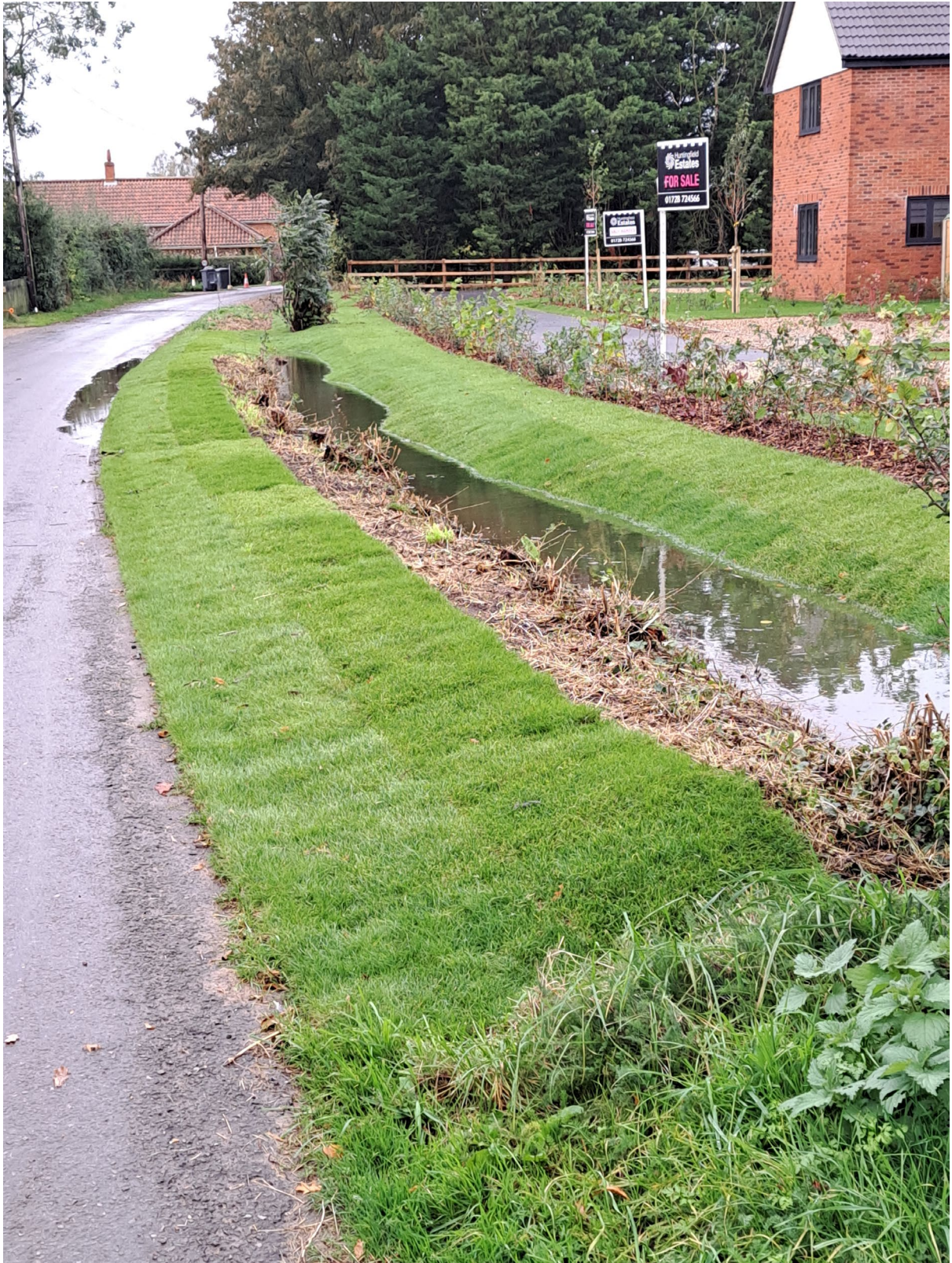
19 October 2023. Ditch nearly full and road surface water draining very slowly.
